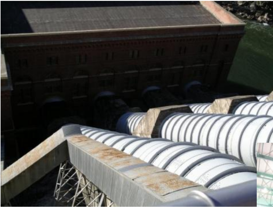
Upper portion of penstock entering powerhouse
