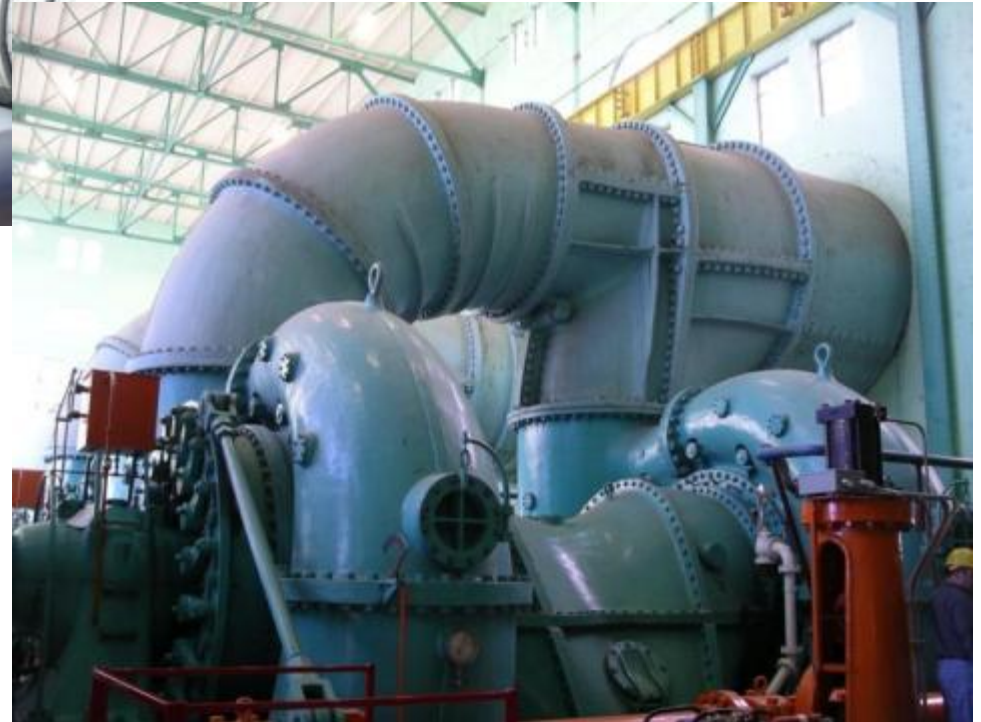
Penstock, scroll cases (housing turbines), and draft chest
